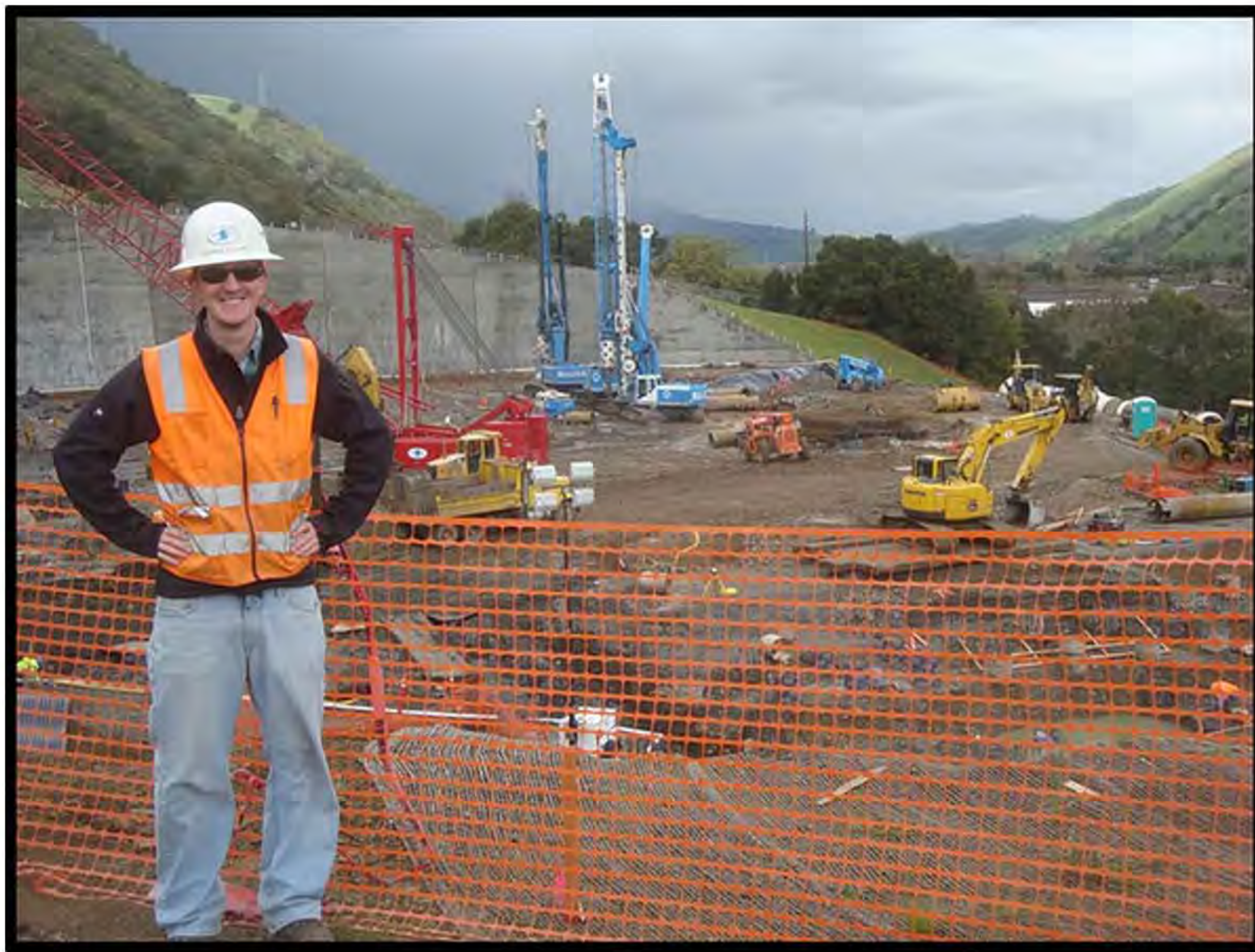
Paul working on a jobsite as part of the Shimmick team
